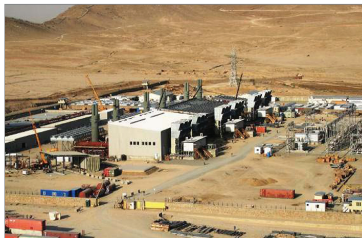
Kabul Power Plant, Afghanistan, 2010. (SIGAR photo)
